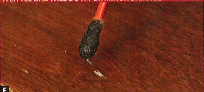
F A dab of stain provides an economical way to cover up light damage. You can also buy scratch cover-up pens at many home centers.
