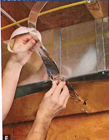
E Apply self-adhesive foil tape along joints in ductwork. Wipe the duct clean so the tape sticks, and smooth the edges to the metal.
