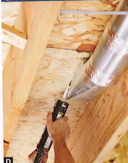
D Seal gaps where heating ducts, water pipes, or other items penetrate walls and ceilings shared with living spaces.
