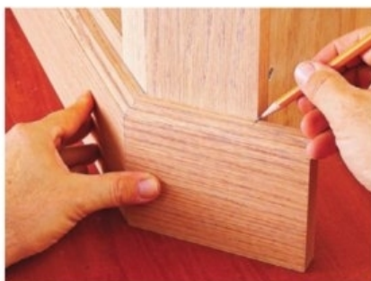
Sometimes it's better not to measure. To determine the length of this trim piece, hold it in position and mark the cut precisely.
