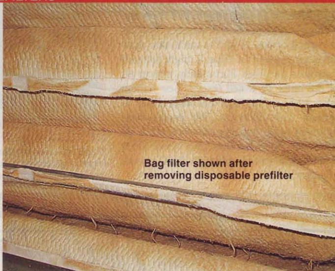
Bag filter shown after removing washable prefilter
