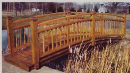
Paul Wiggins of Mount Vernon, Ohio, went to great lengths—16' to be exact—to customize the bridge that now allows access to a small island in his pond. He beefed up the beams, used wood spindles, and made the bridge wide enough to handle his riding mower.
