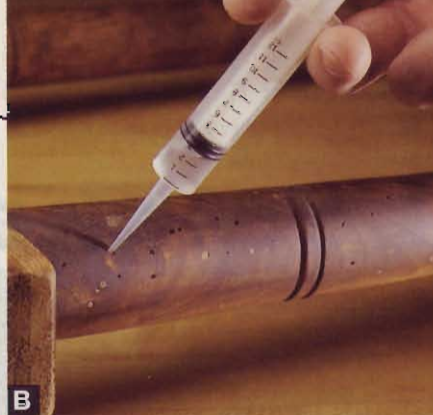
B The surest way to get Bora-Care inside finished wood is to inject it into the flight holes with a syringe. From there it can soak throughout the area.
