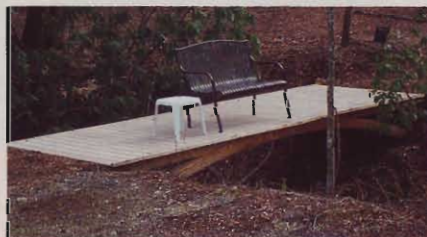
Bill O'Connor of Horse Shoe, North Carolina, wanted a flat-topped bridge across his creek, so he built the 16' arched beams based on our design and attached them to concrete piers on each bank. Bill topped the deck with composite wood planks. Railings are yet to come.
