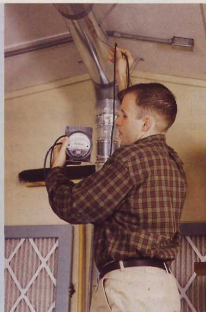
Jeff Hill inserts a pitot tube into the main duct to measure airflow. Opening various gates allows whole-system readings from one location.
