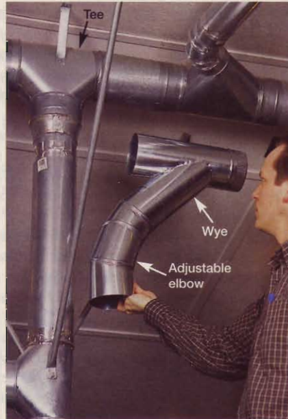
Compared to the tee (installed), a wye and adjustable elbow provide smoother transition from a branch to the main duct.
