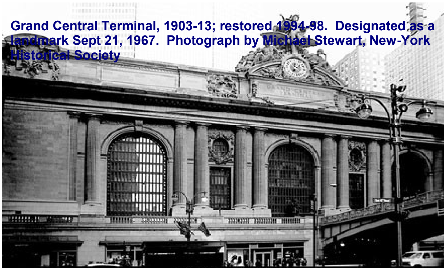
Grand Central Terminal Reed & Stem and Warren & Wetmore, completed 1913
